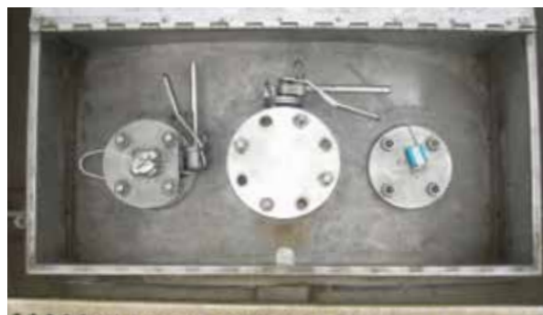
Figure 7: Container Top Connections, DN50 and DN80
